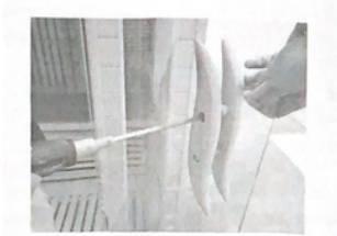
FIGURE 17 INSTALLING THE DOOR HANDLE
