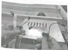
FIGURE 12. MAKE SURE WIRES WERE COLLECTED AND READY TO CONNECT
