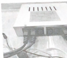
FIGURE 14. PUT DOWN THE WIRES INTO THE SAUNA CABIN
